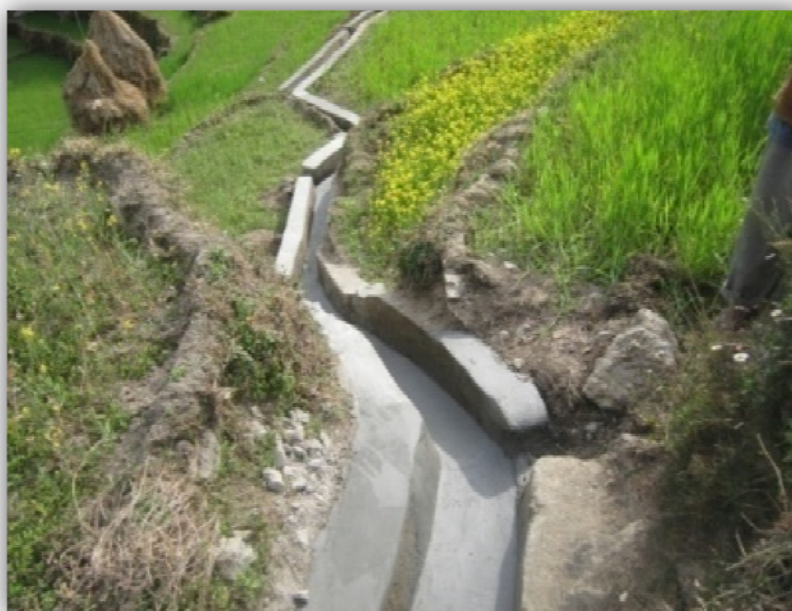
Irrigation guhl constructed under SML in Jolagad cluster (Ukd)
