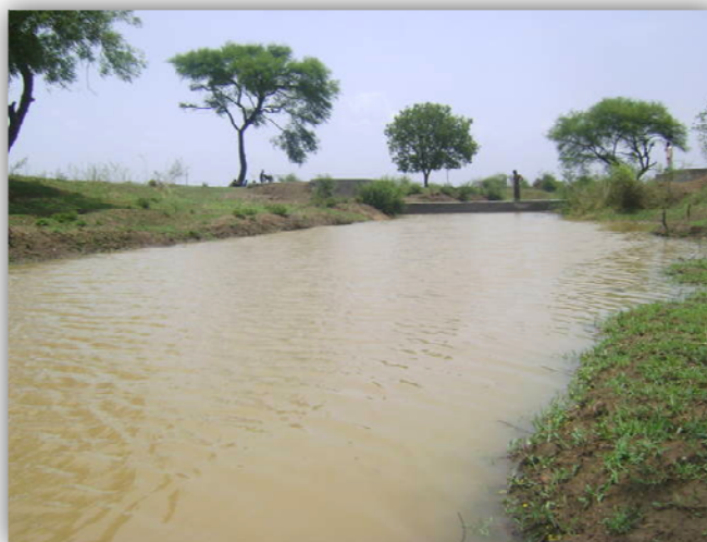
A small check dam in Ghusar village, Akola
