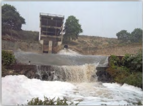
Mixed sewage discharge from Bakshi STP, 1.5 Km upstream of Sangam
