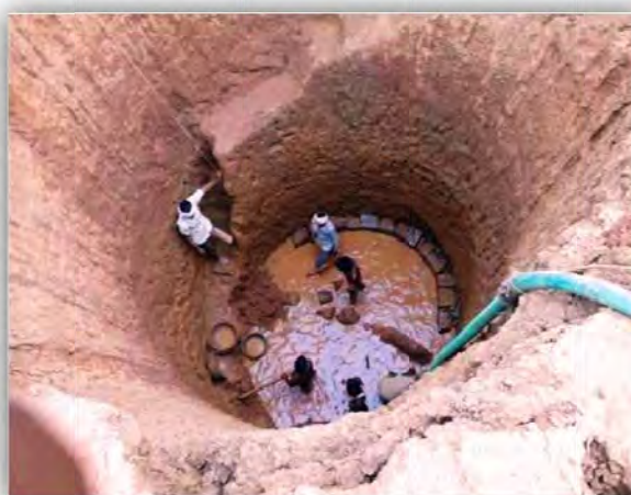
Construction of drinking water well in Birampura village
