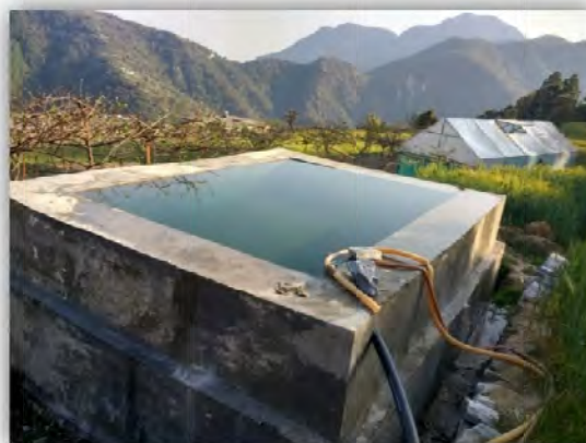
Irrigation tank in Sama village
