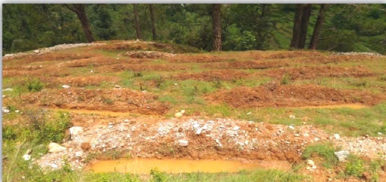
Recharge zone treatment at Jugga Pani source in Siri village
