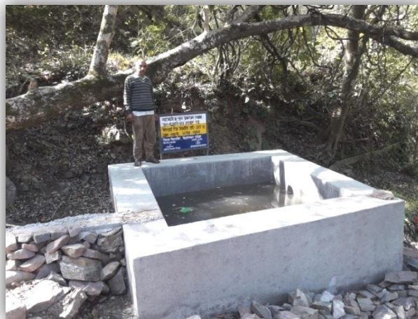
Irrigation Tank Constructed in Luhali Village
