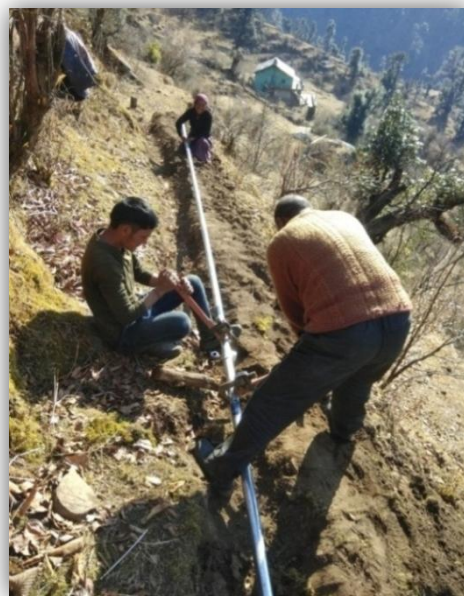
Digging for laying and fitting of pipelines in village Khati
