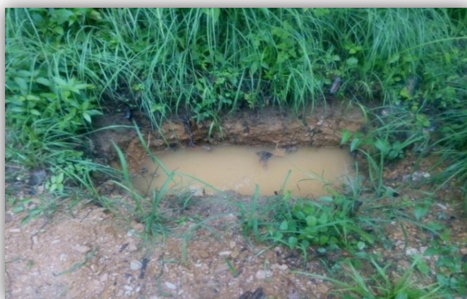
Treatment work for recharge of springs in Rupail
