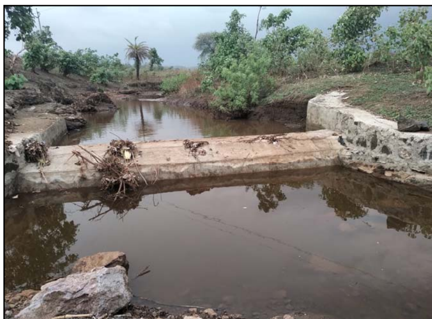
Figure 10: A weir constructed in Jamniamota village, Dhar
