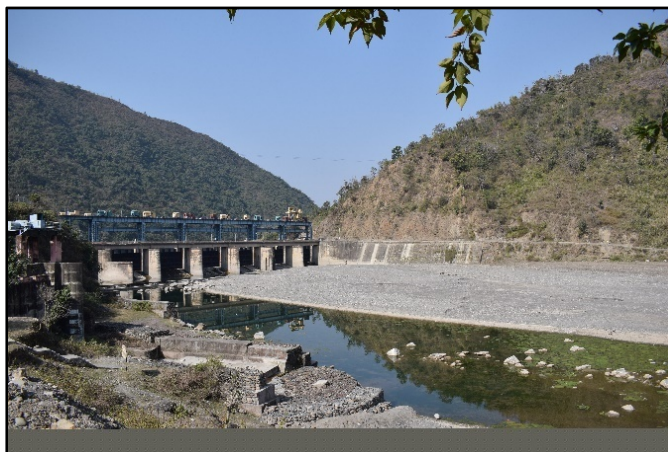
Giri Project, downstream of diversion
