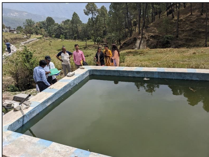
Storage tank for irrigation in Khirganga project, Kapkot, Bageshwar
