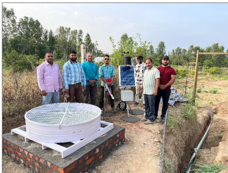
Installation of Automatic Weather Station at GFIC
