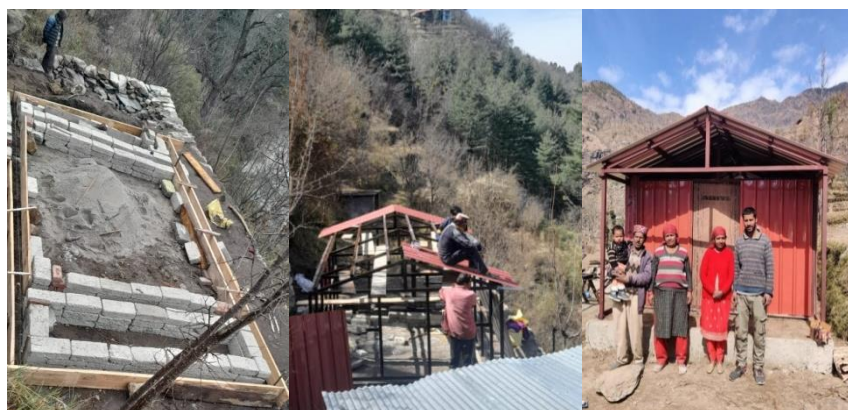
Construction of Temporary Shelter
