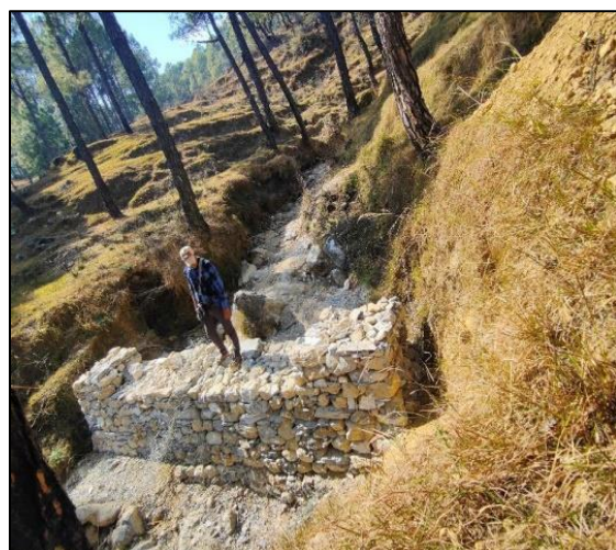
Gabion Check Dams (GCD) Construction of for reducing the velocity of water of stream, it also helps in storage of water, recharge of spring, and irrigation.
