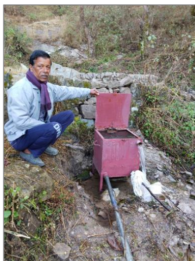
Construction of storage tank for and 88m drinking water pipeline
