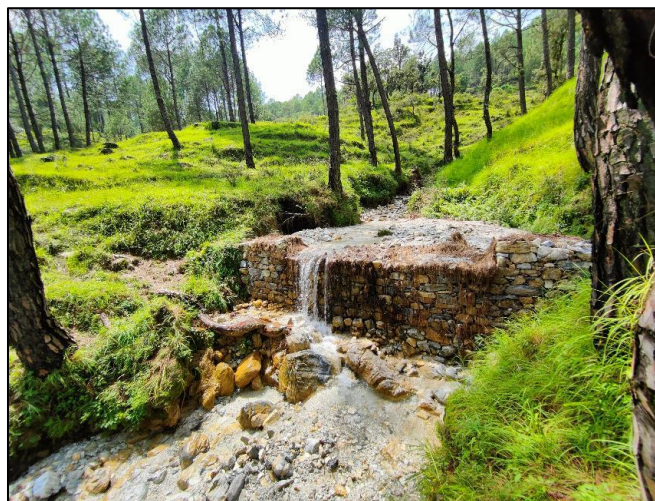
Gabion Check Dams (GCD) Construction of for reducing the velocity of water of stream, it also helps in storage of water, recharge of spring, and irrigation.
