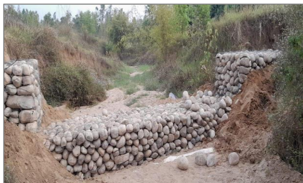
Construction of Gabion
