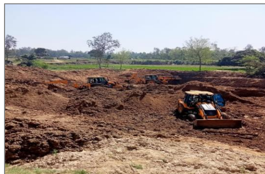
Excavation of soil
