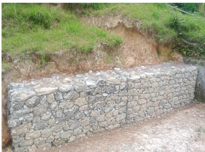
Gabion retaining wall village Malladesh
