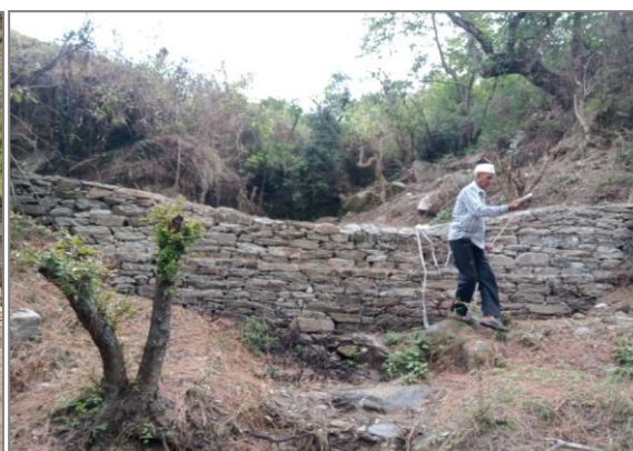
Gabion retaining wall for the protection from soil erosion and water conservation
