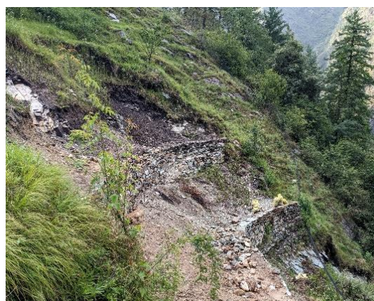
Protection walls for soil conservation
