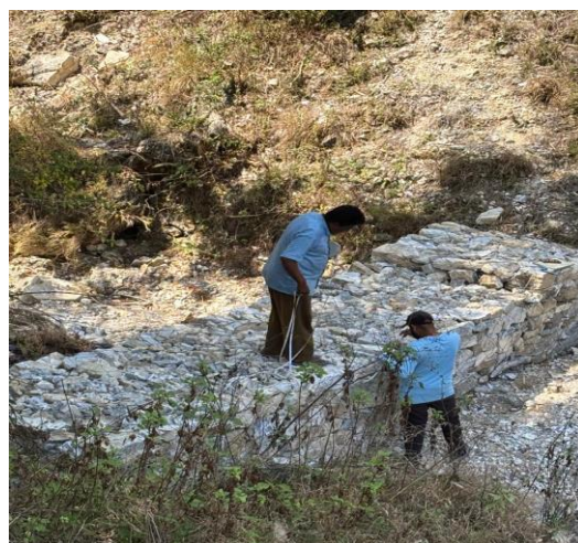
Gabion check dam for soil and water conservation village Farsali
