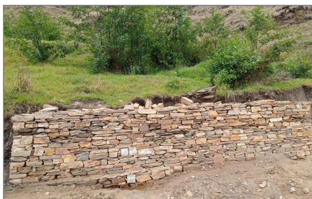
Retaining wall dry for the protection from soil erosion and landside
